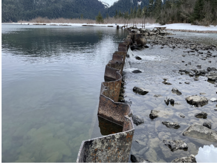
FIGURE: Crest of Eyak Weir
