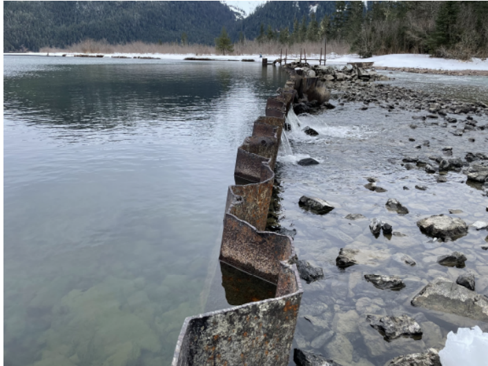
FIGURE: Crest of Eyak Weir
