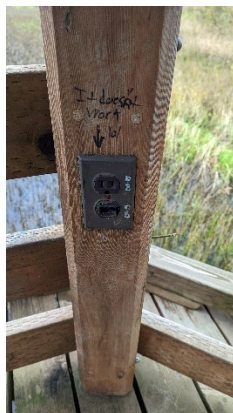
Fig. 14. Damaged Unpowered Receptacle at Gazebo
