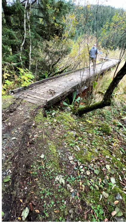
Fig. 1. Gravel and termination at boardwalk
