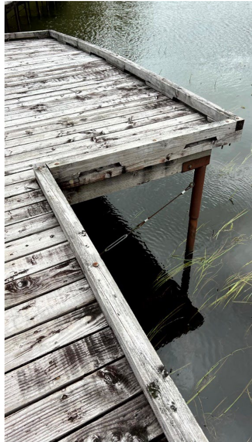
Fig. 11. Sagging Boardwalk at Southern Widened
