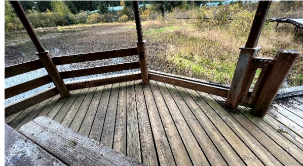
Fig. 13. Gazebo Missing Guard Beams
