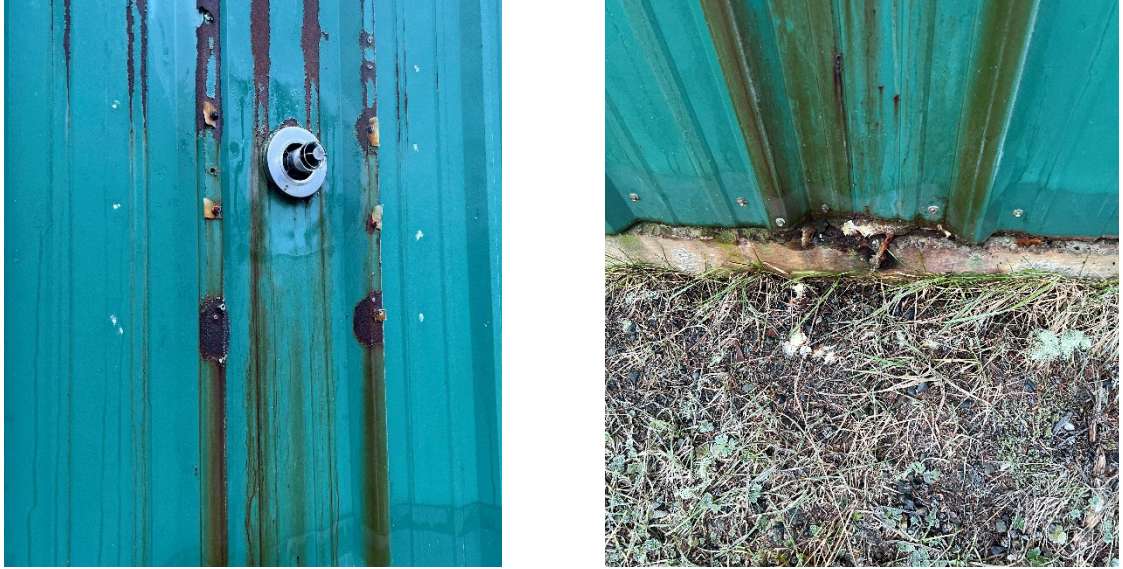
Fig. 5. Missing Heat Deflector and Damage
