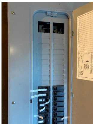
Fig. 23. Main panel with missing circuit breaker covers
