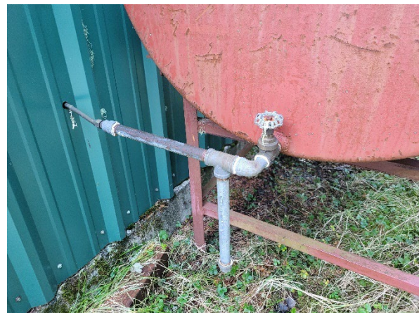
Fig. 18. Fuel piping
