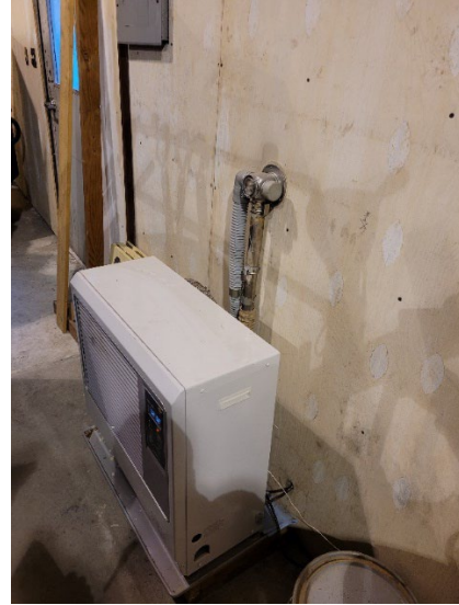
Fig. 16. Evidence of exhasut leak on flue
