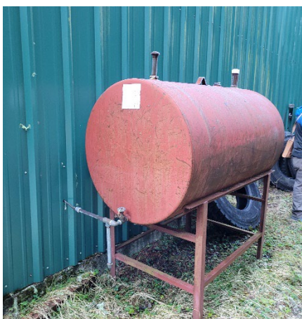
Fig. 19. 300 gallon waste oil tank.
