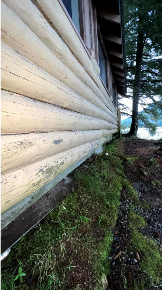
Fig. 9. Lakeside Deteriorated Logs.
