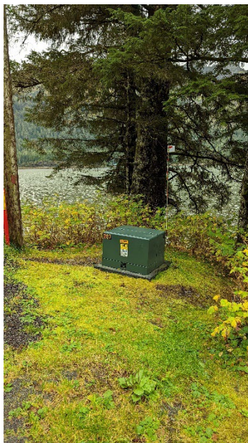
Fig. 17. Service transformer
