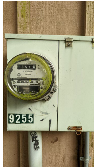
Fig. 16. Electrical Service Combination Meter Main
