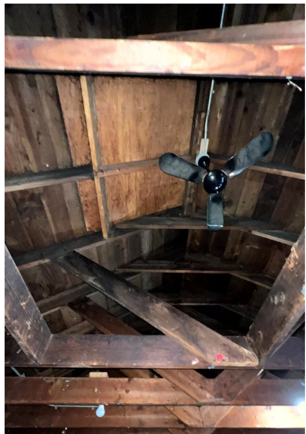
Fig. 8. Altered Roof Trusses
