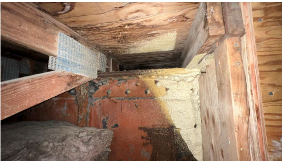
Fig. 16. Original Roof Trusses on Interior Girder
