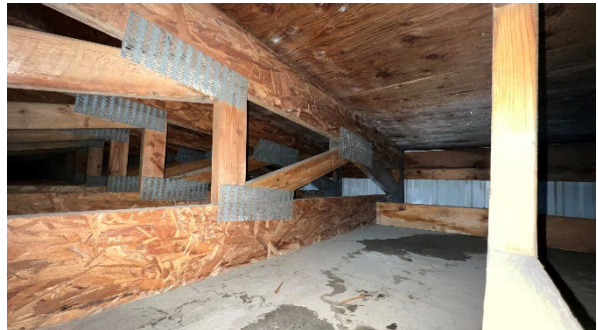
Fig. 17. Overframed Roof Truss Eave End
