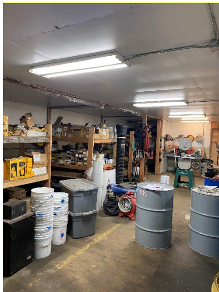
Fig. 45. Fluorescent lights below mezzanine missing lens
