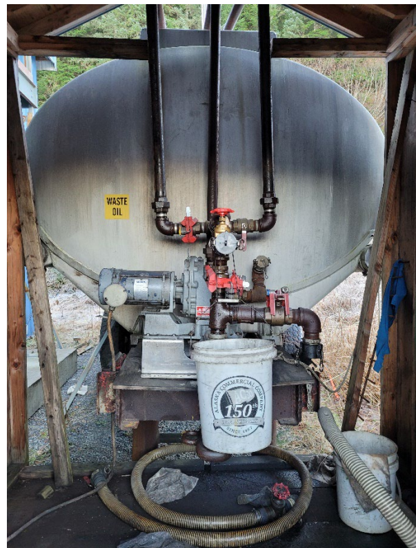
Fig. 32. Waste oil tank and piping
