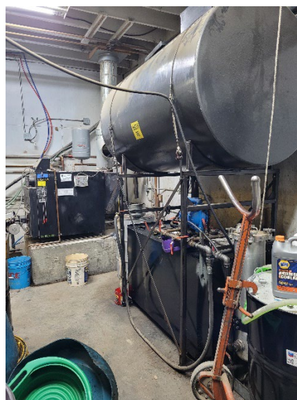
Fig. 40. 500 gallon settling tank and 300 gallon day tank.
