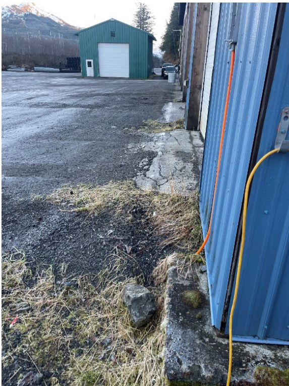
Fig. 19. Concrete apron at bay entrances
