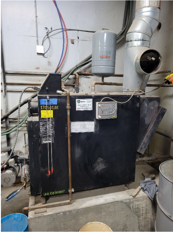
Fig. 25. Multi fuel boiler
