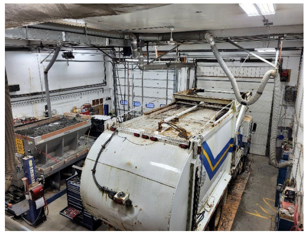
Fig. 24. Main two bays (east end), note vehicle exhaust system
