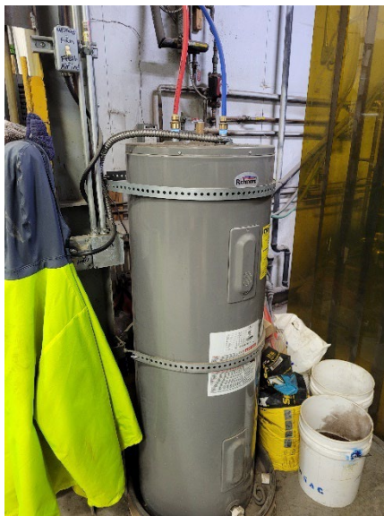
Fig. 37. Electric hot water heater
