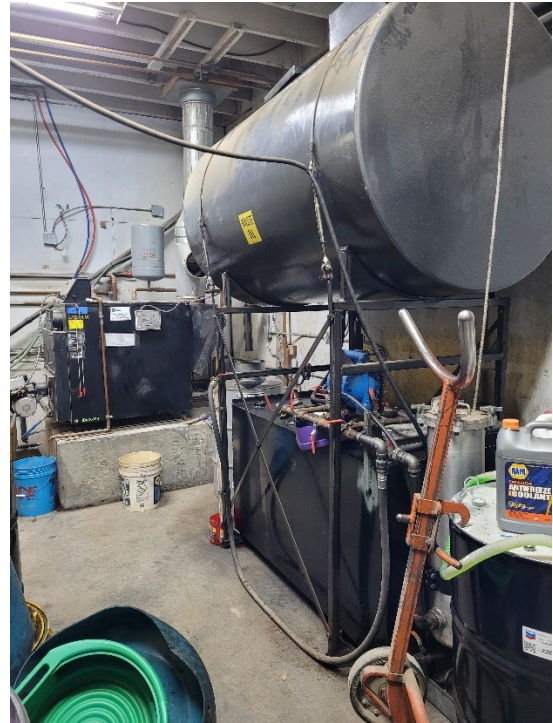
Fig. 22. Oil settling tank with day tank below, boiler in background
