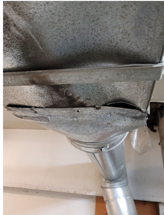
Fig. 28. Damage to vehicle exhasut ductwork
