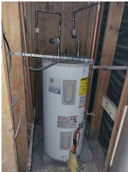
Fig. 15. Electric hot water heater
