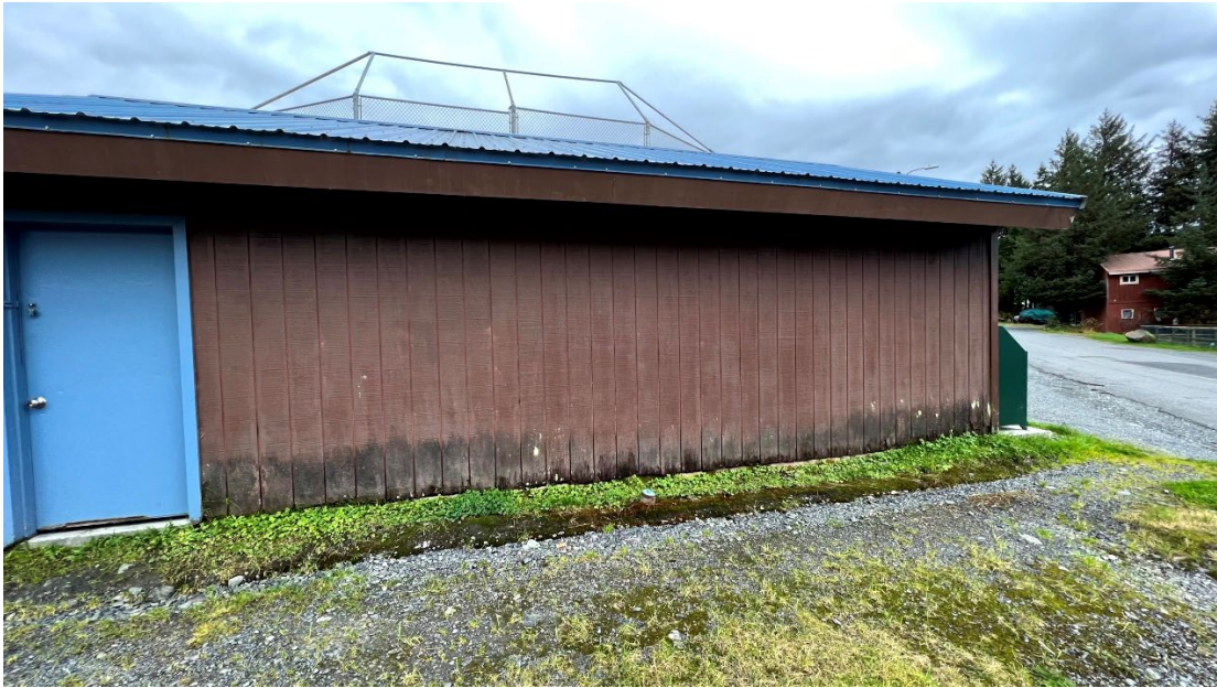
Fig. 1. Visible siding damage at rear elevation
