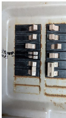
Fig. 19. Branch Circuit Panelboard Interior
