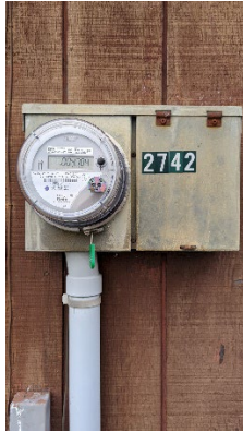
Fig. 17. Electrical Service Meter/Disconnect
