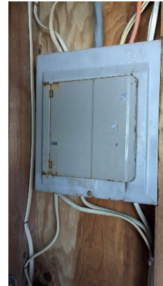
Fig. 18. Branch Circuit Panelboard exposed wiring
