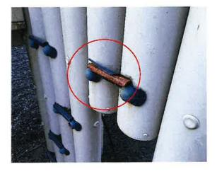
There are connecting points on the structure steppers that are worn to the point of needing to be replaced.
