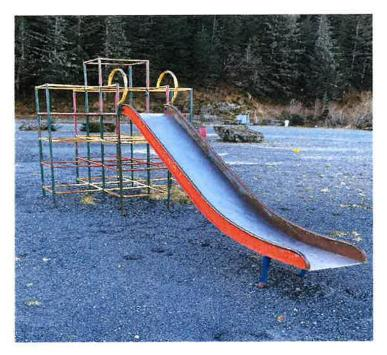
The play structure is a residential structure and does not meet the safety requirements of ASTM 1487 for Public Parks.
