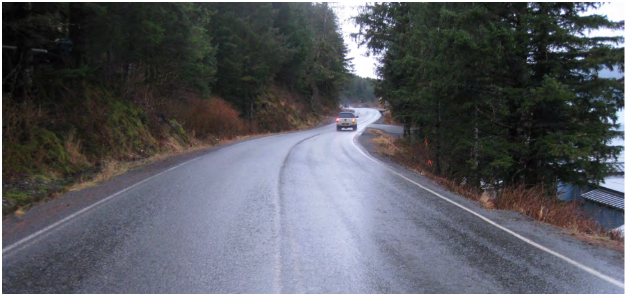
Figure 1: Example mountainous road pavement width with steep topographic features on both sides of the roadway. (source: DOT&PF file photo, Point Whitshed Road MP ~0.4, 2019)
