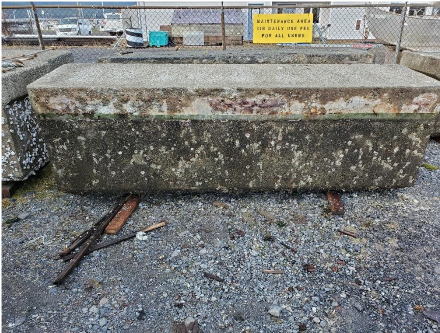
Finger float sections prepped for rebuild
