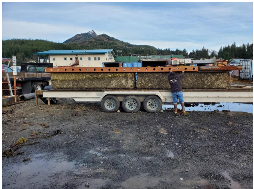
Finger float sections being reassembled with new timbers and fasteners
