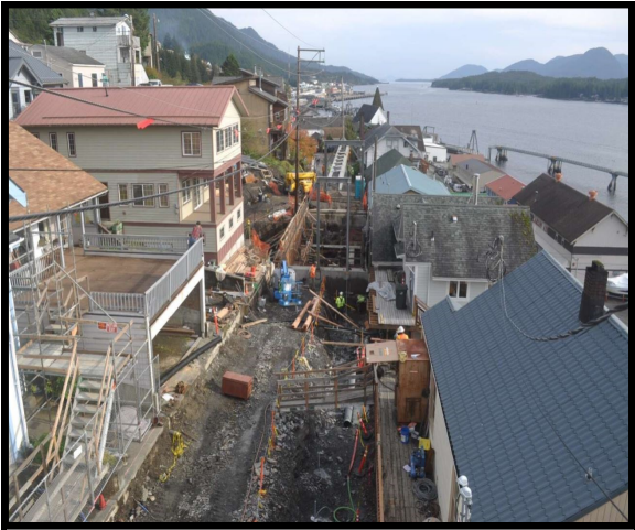
KTN Water St : preparing for the 1st girder launch
