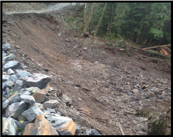
Shelter Cove Rd slope failure after over 2.5 inches of rain in 12 hours.
