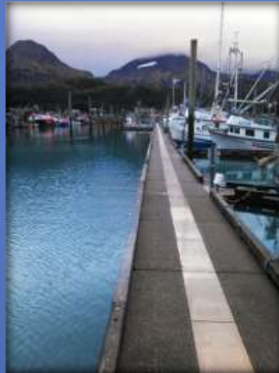
Bull rail replacement
