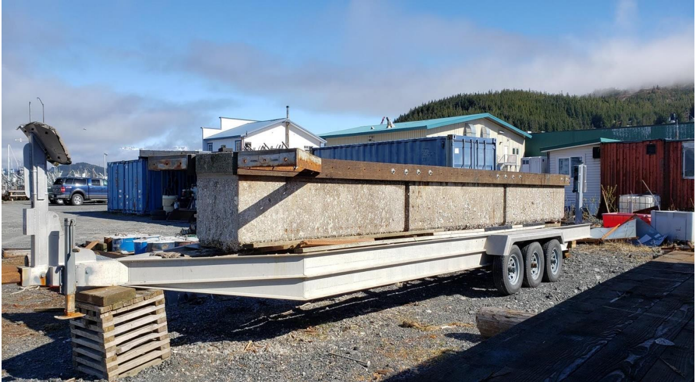
Rebuilt finger from J-float on trailer ready to back in the water
