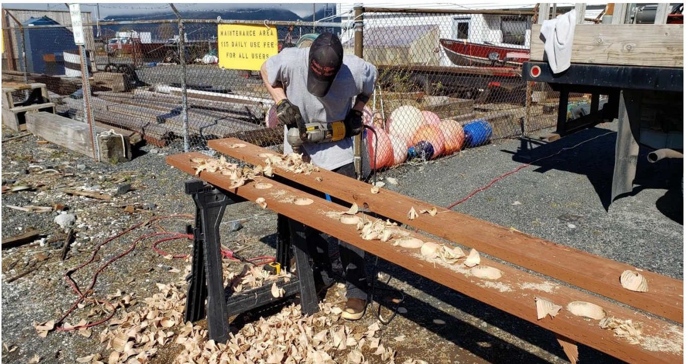
Drilling splash boards for finger float rebuild
