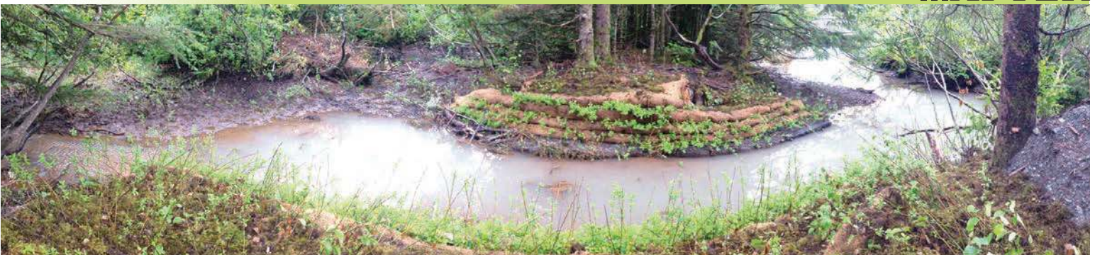
By removing the old culvert the stream is able to flow freely into the pond.
